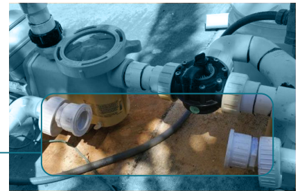
After pipe is cut and unions have been glued in place
