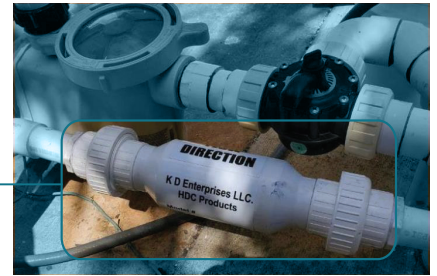
After device is fitted and connections are made
