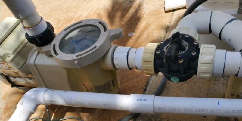
Step 1: Image of plumbing prior to installation, showing a straight run of pipe for device fitment.
